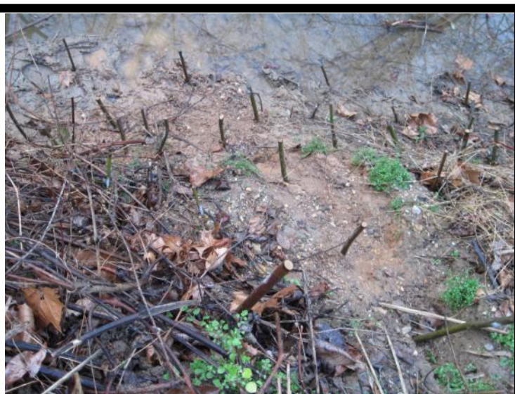
Option 2: Plant diverse, native flora without changing the grade (above left illustration). Above right photo shows livestakes installed every 1' on existing slope to create snag and quick root mass (© N. Alexander).
